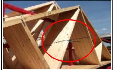
4. On instruction from the site responsible person the driver will release the transport straps on the side being unloaded ensuring no one is within the danger area as shown in the pics 5—8.
