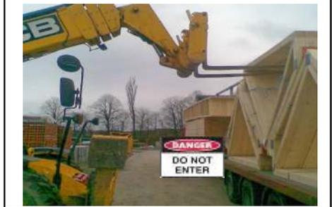
7. The driver will cut the individual rope attaching the pack to the bars. This must be carried out from a safe position using the drivers cutting tool.
