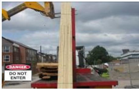
6. **NEVER** stand between the forklift and trailer, do not allow others to enter this danger area. **NEVER** stand on or under the forks. Ensure the danger area remains clear at all times.
