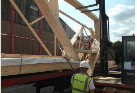
8. The forklift truck operator must lift the trusses from the trailer and then follow his company training and offloading procedures to revert the trusses.
