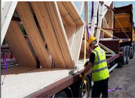
5. Once the order of unloading is agreed between the slinger and driver the slinger will attach the purple lifting slings to the crane hooks.
