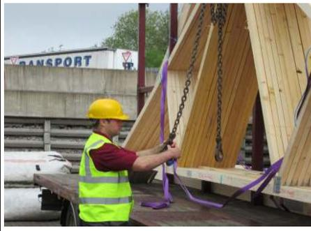
6. The crane will then take up the slack of the lift prior to the rope being cut.
